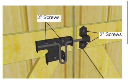
**67.** Attach Black Barrel Bolt as illustrated above with 2" & 3/4" Black Screws. Note how female part of Barrel Bolt is positioned higher than male. Do a dry run first to position Barrel Bolt correctly. **Important** - Drill a shallow pilot hole with 1/8" drill bit prior to securing with screws to prevent wood splitting.
