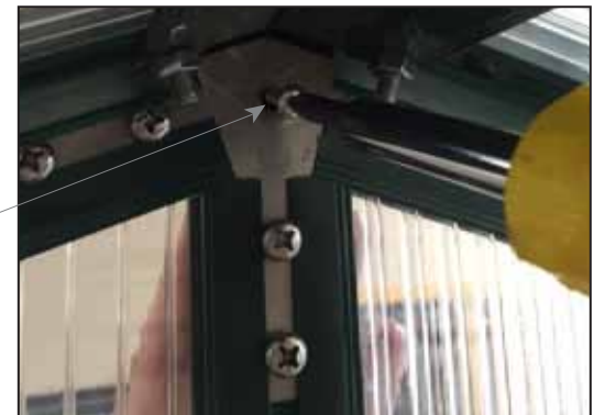
Interior greenhouse view of mid roof cap, where Z06 screw goes through WG01 mid hole into the end cap.
