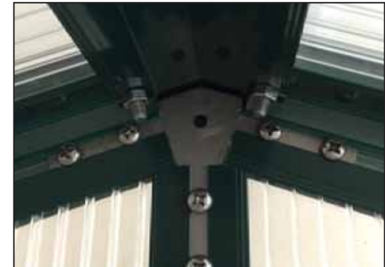
Interior greenhouse view of mid roof cap, where Z06 screw goes through WG01 mid hole into the end cap.
